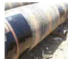
Floating hose repair
