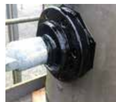
Transformer leak sealing
